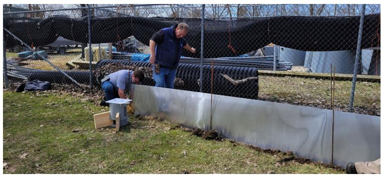
7. Place the bucket so that it is flush with the fence and the ground. Drill two small holes in the front of the bucket on either side of the fence.
