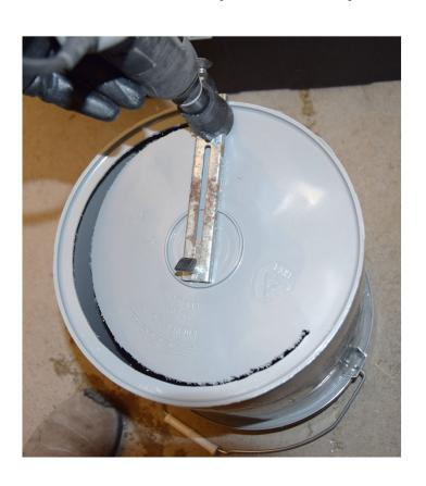
2. Identify and mark a center point, between the bucket handle attachment points. Wrap measuring tape around bucket, beginning on this center point, and mark:
